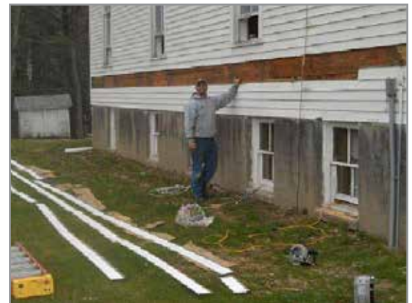
Kyle Williams from Shoemaker Cos. updating electrical wiring
