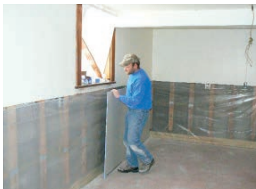
Drywalling basement walls
